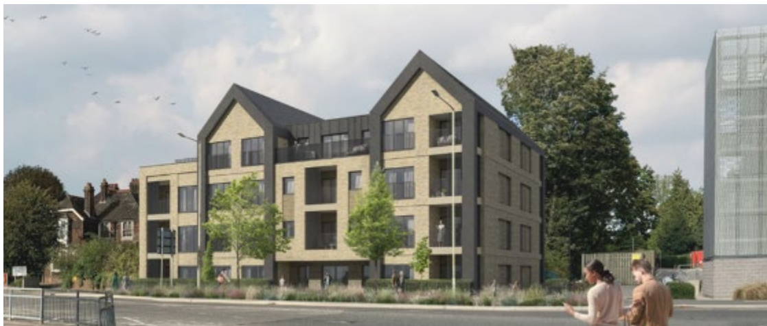
Figure 5: view of apartment block facing Elwick Road
