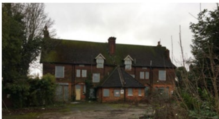
Figure 2: Rear of Swanton House
